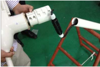
Pass the wire through the pole.
